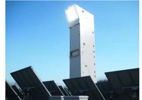
Solar Tower (Central Receiver System)
